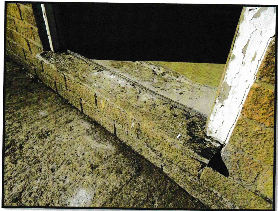
Fig. 26. External timber threshold and door frame are worn.
