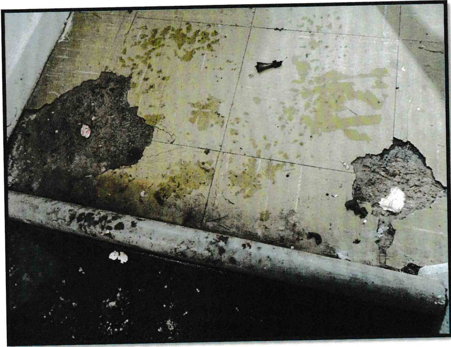
Fig. 51. Damaged vinyl floor tiles in the changing rooms.
