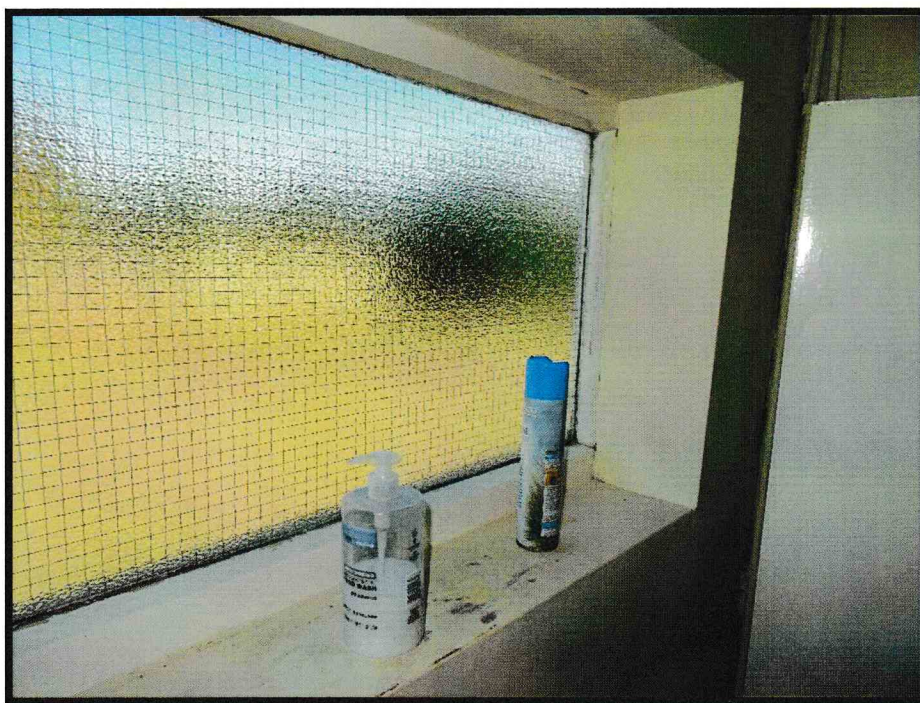
Fig. 40. Dilapidated finishes to the ladies toilet window cill
