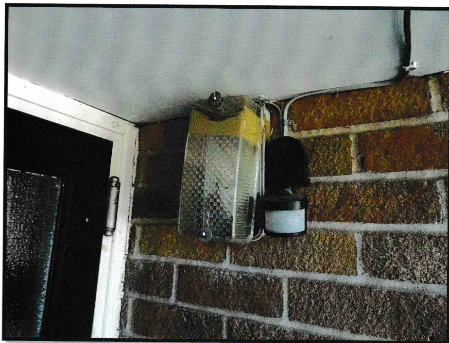
Fig. 12. Damaged external lobby light fitting
