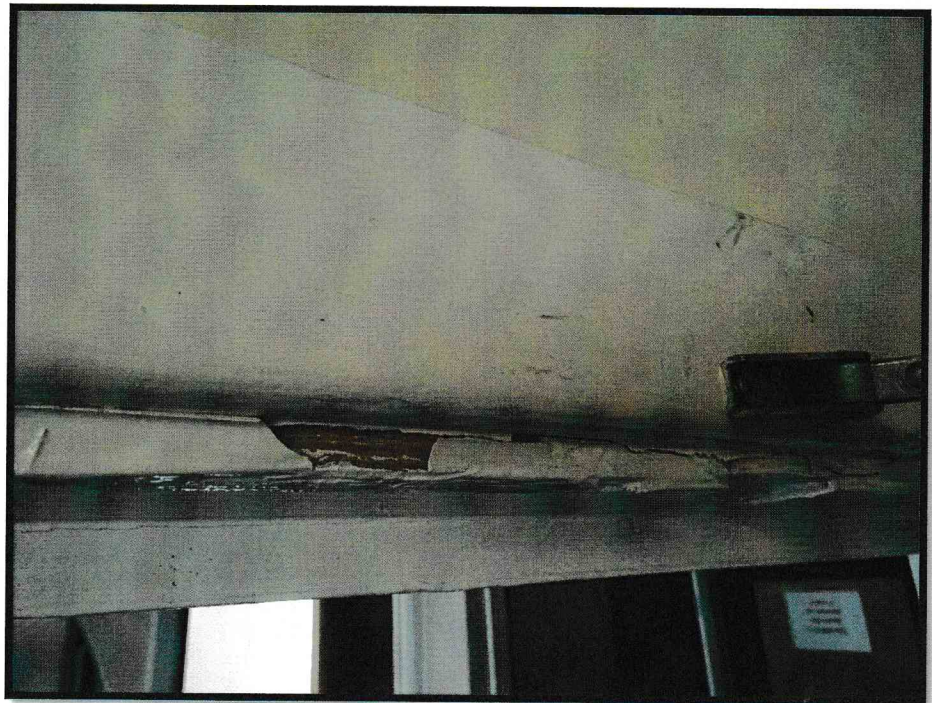
Fig. 38. Damage to the head of the kitchen door
