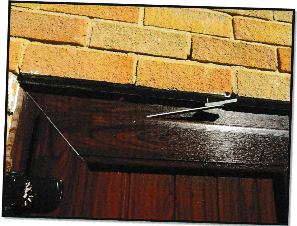
Fig. 17. Damaged door closer arm requires attention
