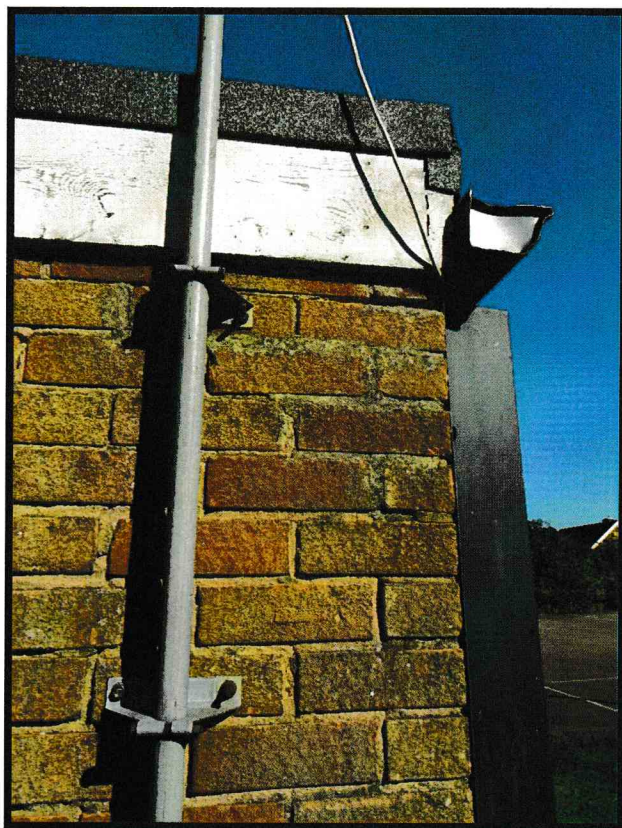
Fig. 15. Minor cracking on the mortar joints to the external corner
