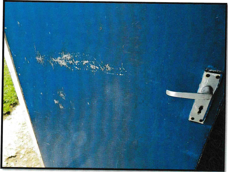
Fig. 25. Changing room doors require redecoration and replacement ironmongery
