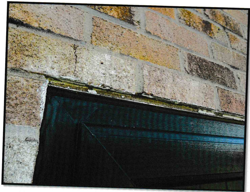
Fig. 05. External door head requires minor making good
