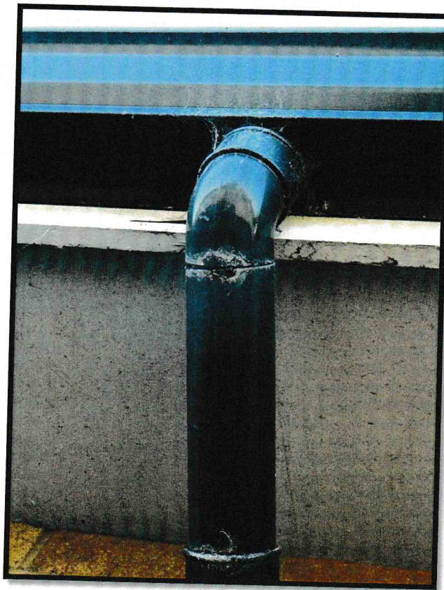
Fig. 10. Rainwater pipe joints starting to leak slightly
