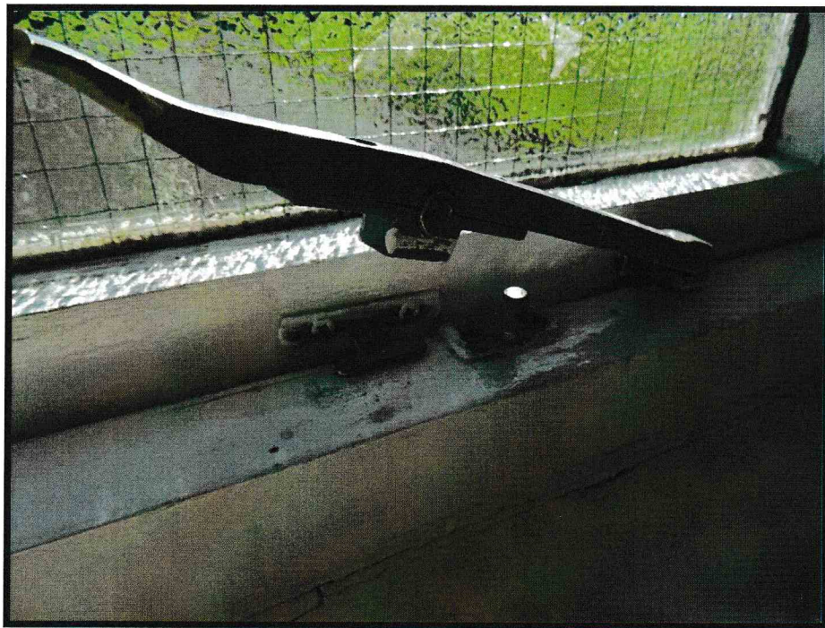
Fig. 45. Inoperative lock to the window in the gents toilets
