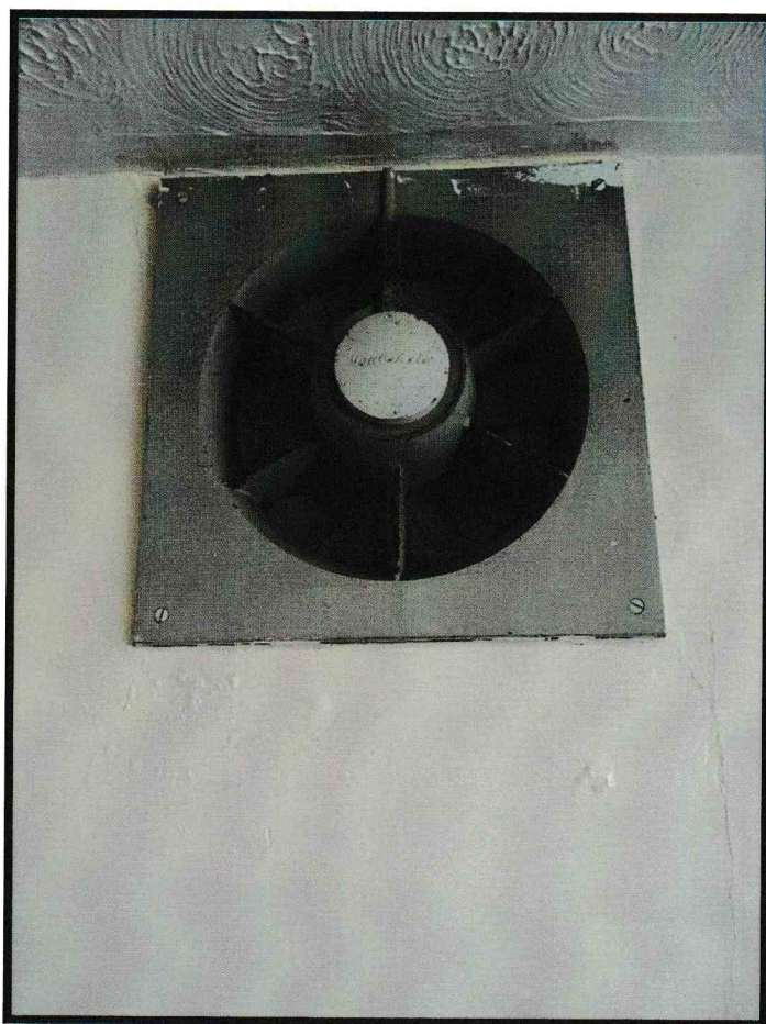
Fig. 36. Kitchen extract fan, note minor damp evidence in the wall below
