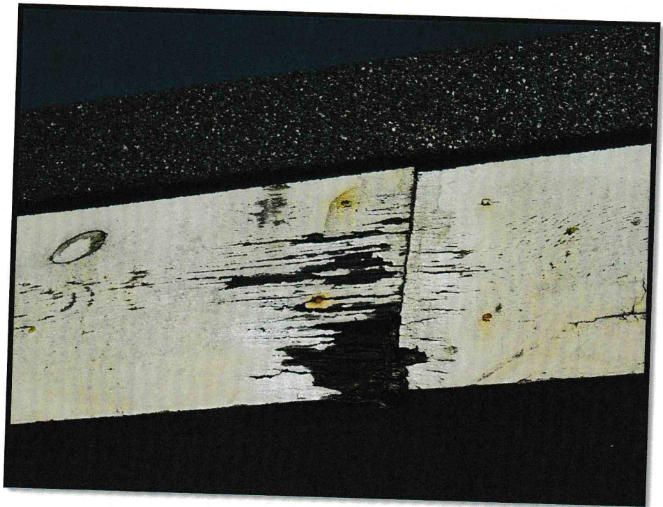
Fig. 18. Further rotting to the fascia boards to the rear of the building
