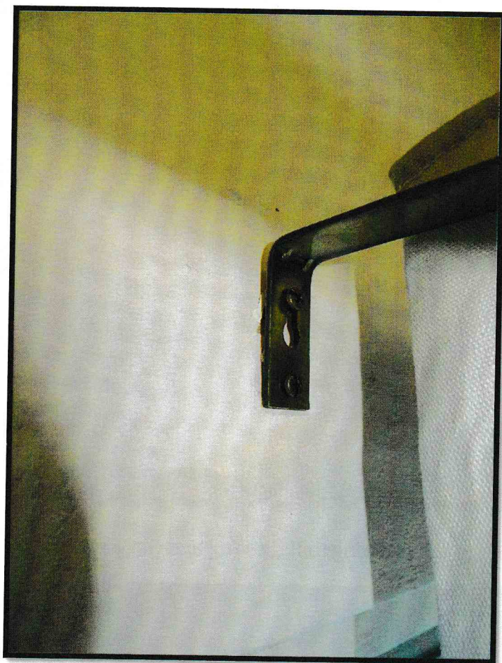
Fig. 31. Curtain rail fixing requires tightening
