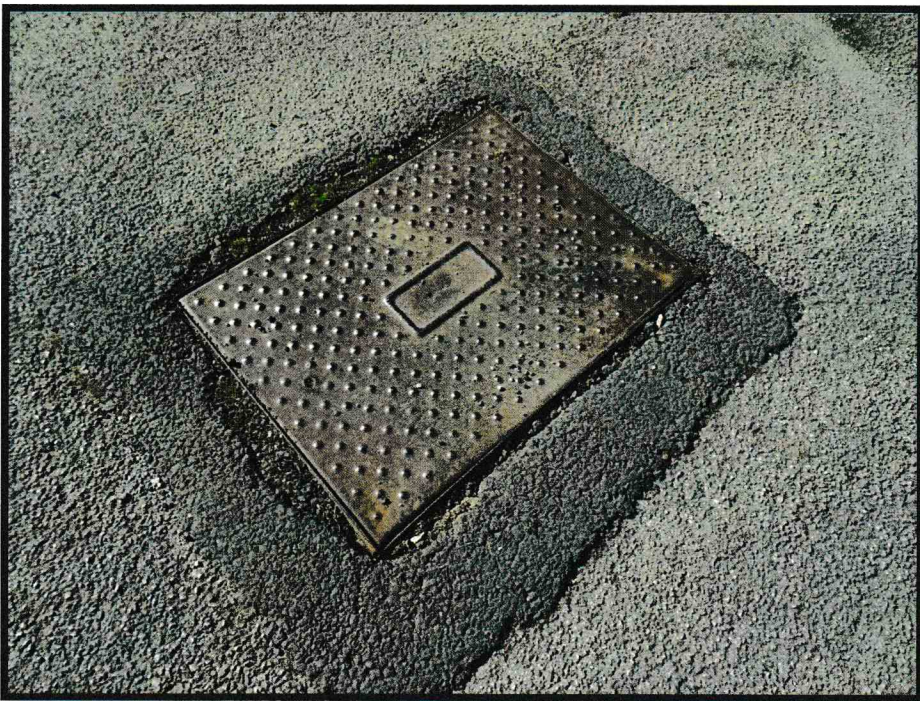
Fig. 28. Manhole cover specification should be checked for strength
