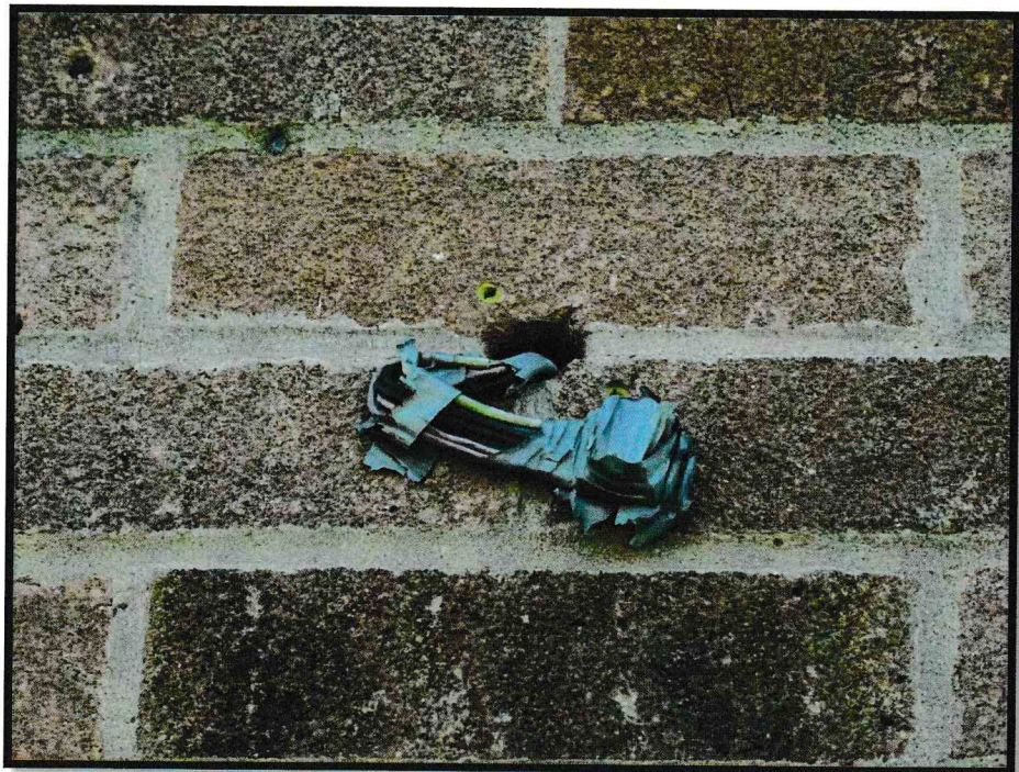
Fig. 14. Cables requiring proper termination
