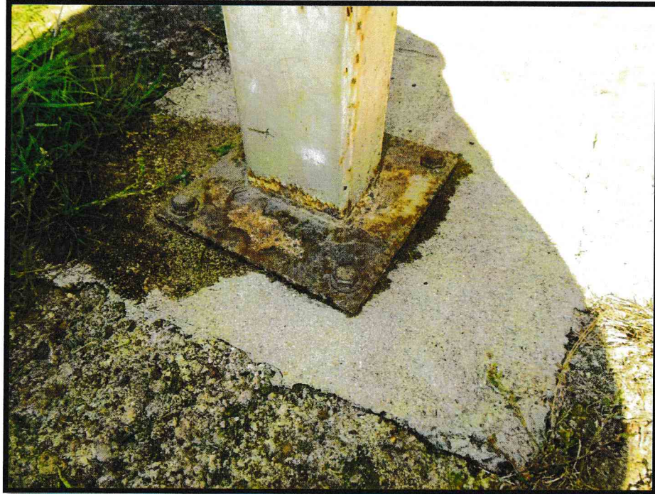
Fig. 21. Corroded canopy post foot, water on ground suggests gutter stop end leaking
