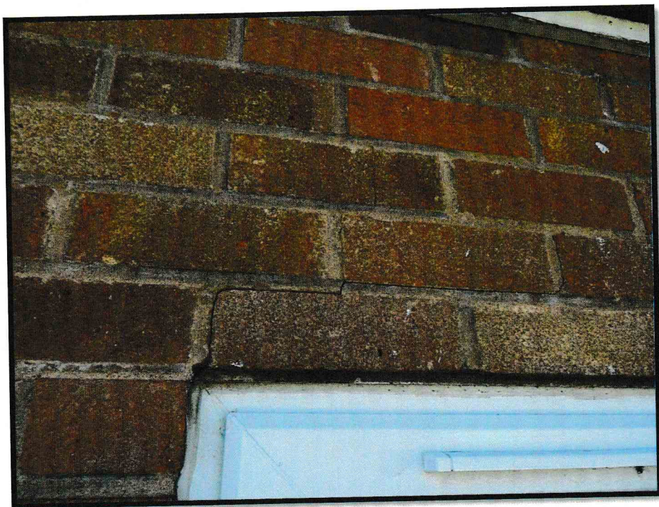
Fig. 01. Minor settlement crack above window lintel
