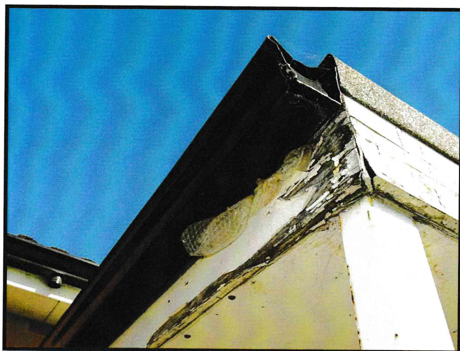
Fig. 20. Damaged fascia to the external canopy at the rear
