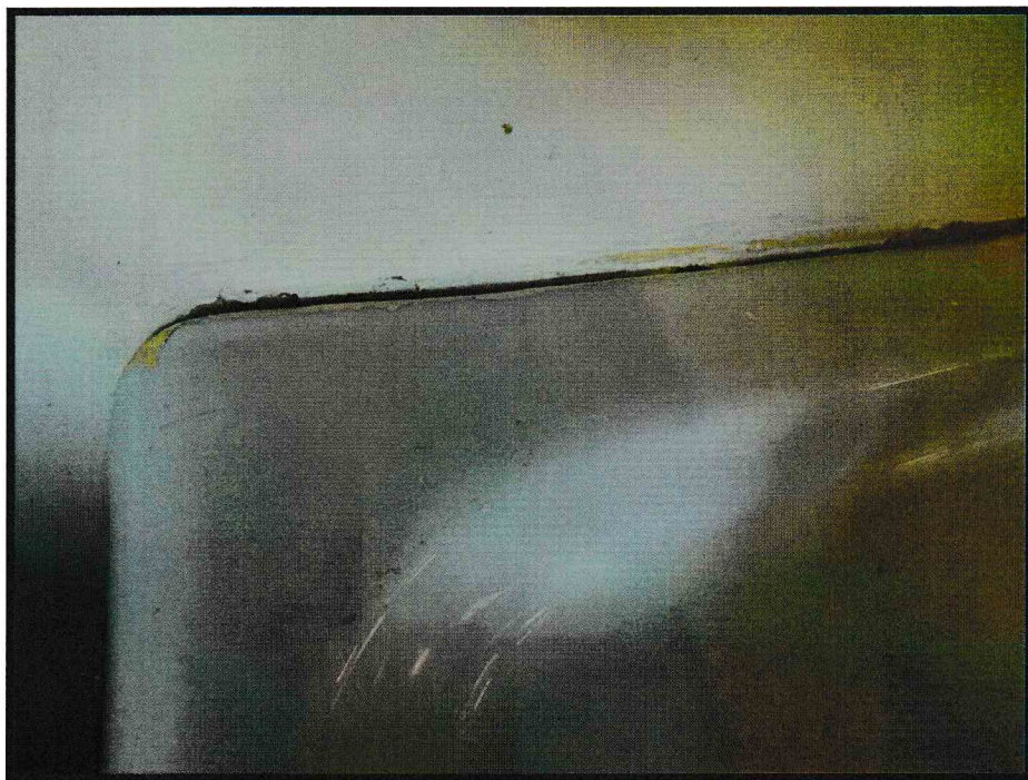
Fig. 39. Gap to the rear of the kitchen wash hand basin
