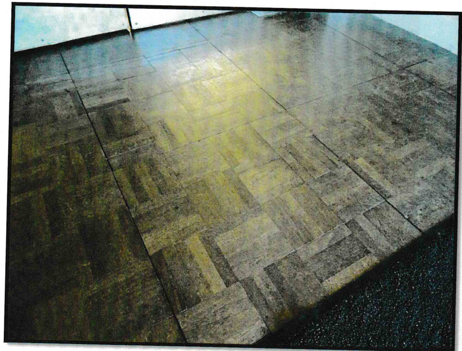
Fig. 34. The timber parquet flooring panels
