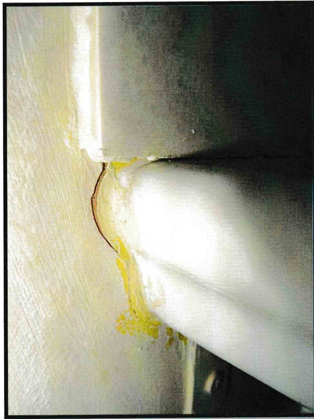
Fig. 41. The basin in the ladies toilet which is loose on the wall
