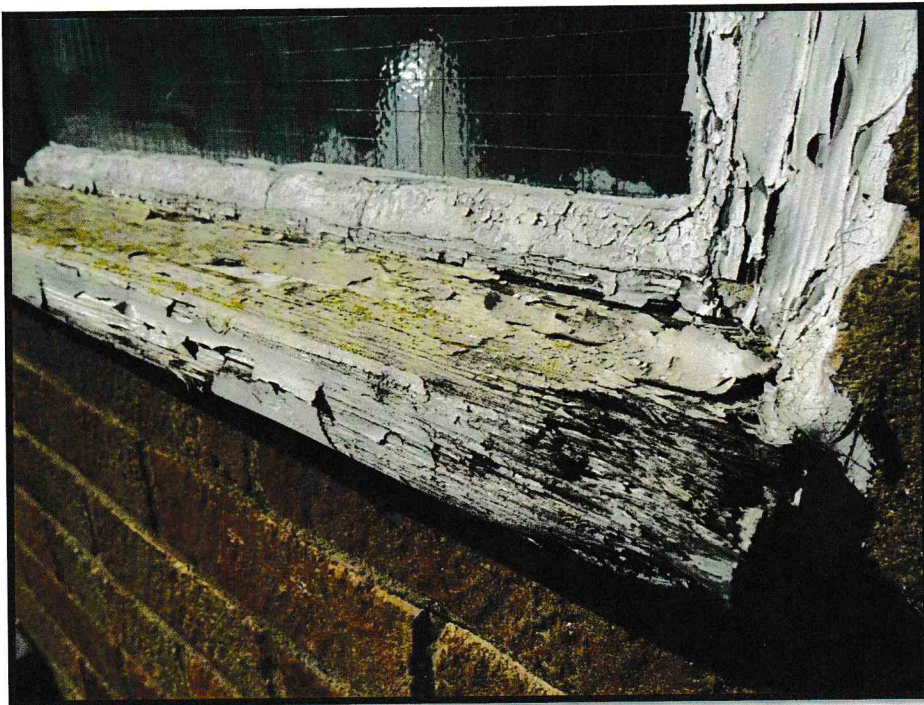
Fig. 24. Rotten external timber window frame and cill
